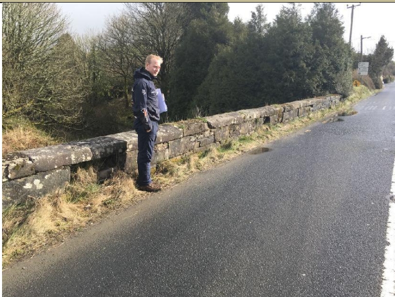
Figure 8: Showing the existing low parapet wall on Anglesey Bridge. Note lost ashlar
